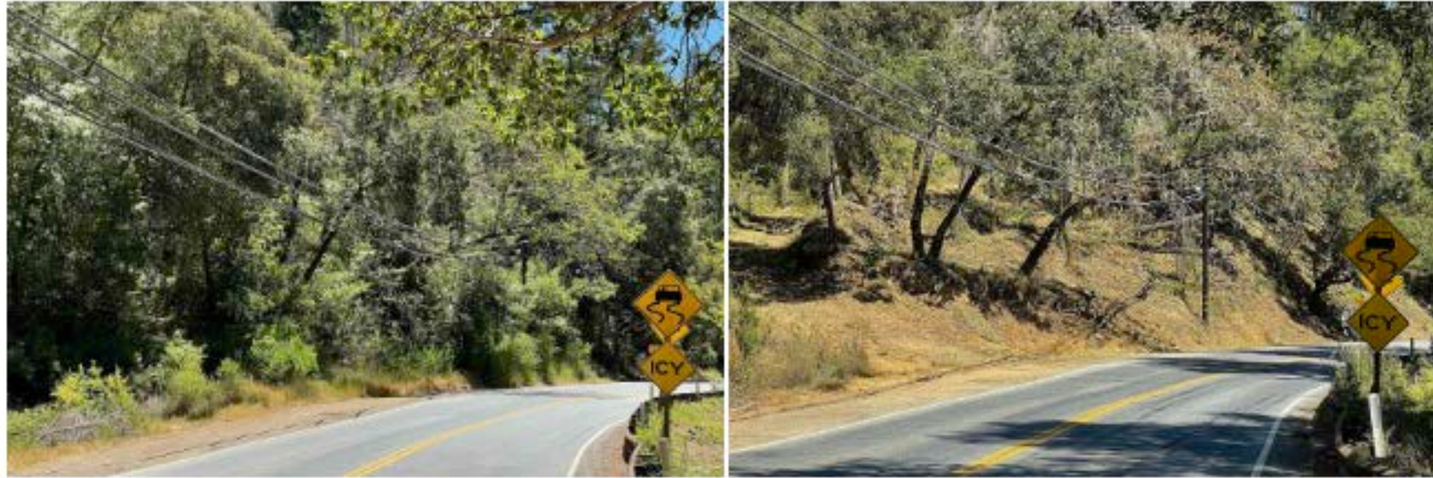
Photos: Before and after shaded fuel Break work on Summit Road.
